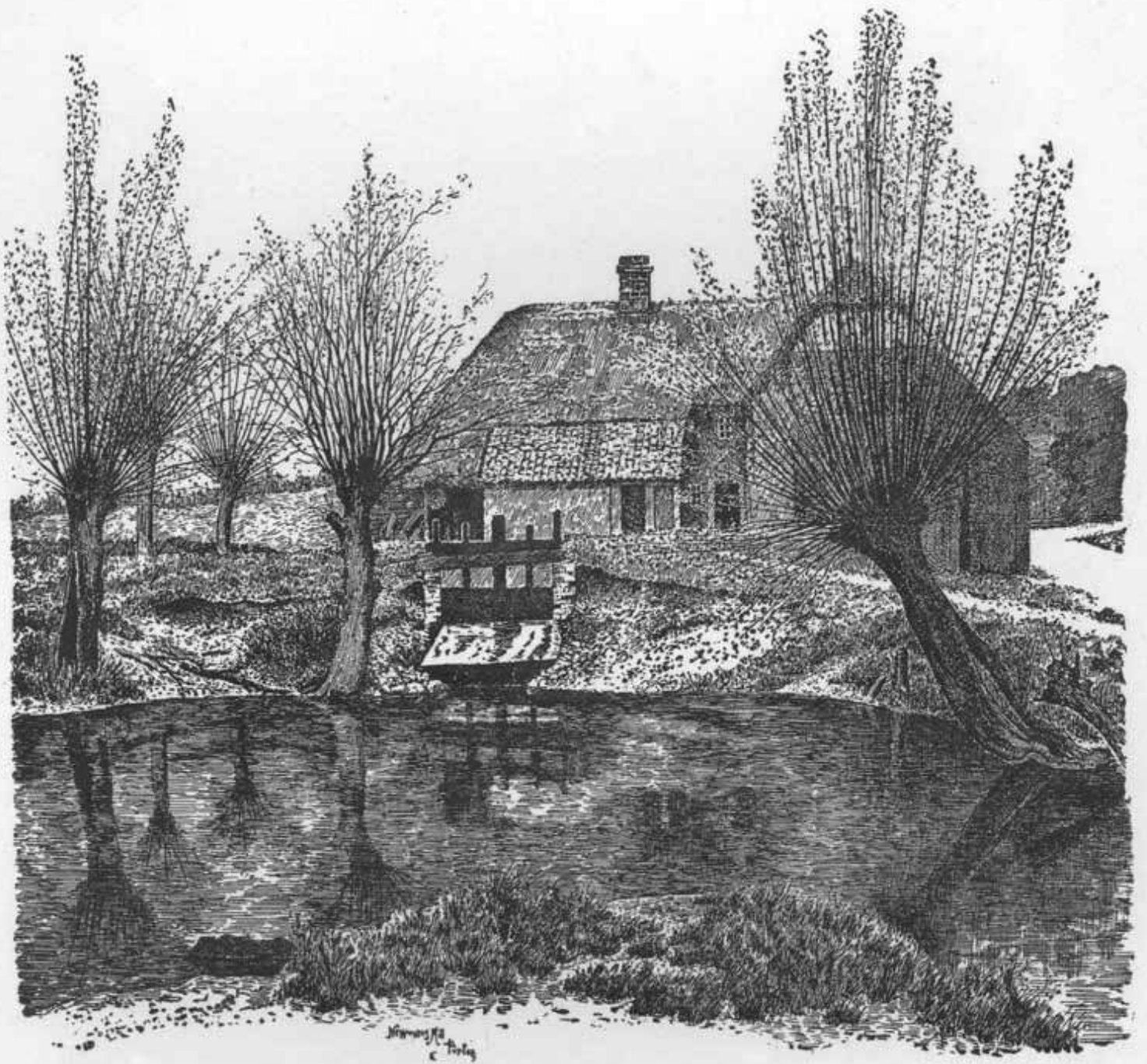
Newman's Mill, formerly the Ridgeway Mill.
