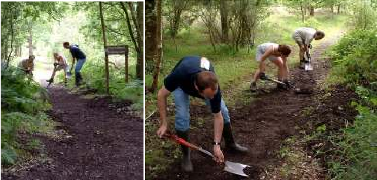
Above – Phil, Caragh, & Ben clearing the footpath.
