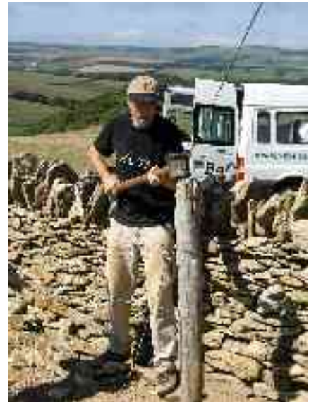
Top - Richard & Mark working on the coping stones Above - David knocking in a stake for the barbed wire fence.
