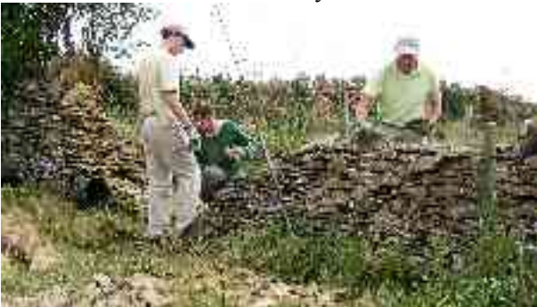
David, Laurence & Maurice demolishing the wall
