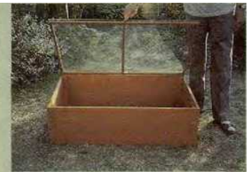
4. Connect the battens with angle brackets, attach plastic cover and fix to base with hinges
