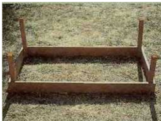
1. Screw the bottom rails to the posts using brass or zinc-coated screws
