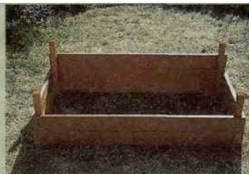
2. Build up the base, making sure there are no gaps for draughts to penetrate
