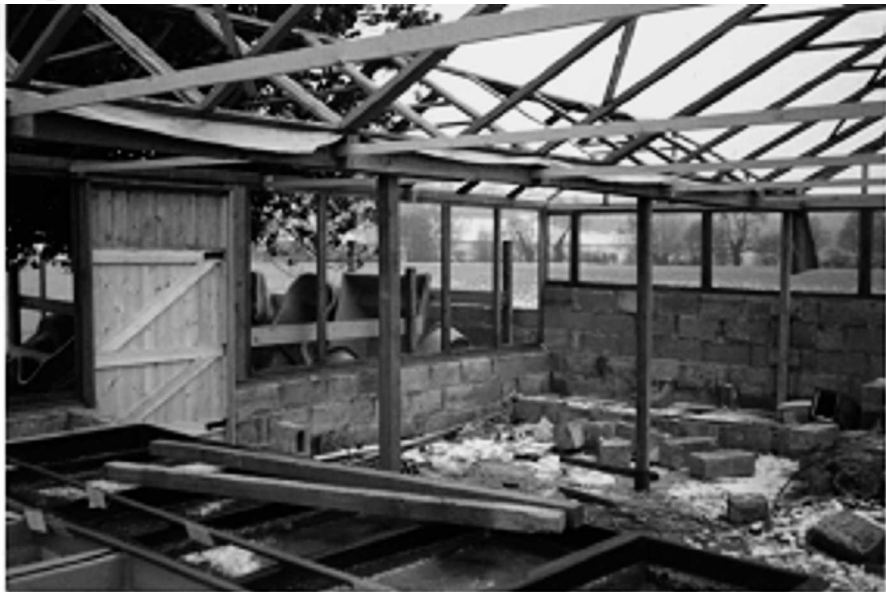
The New Fish department Under Construction.
