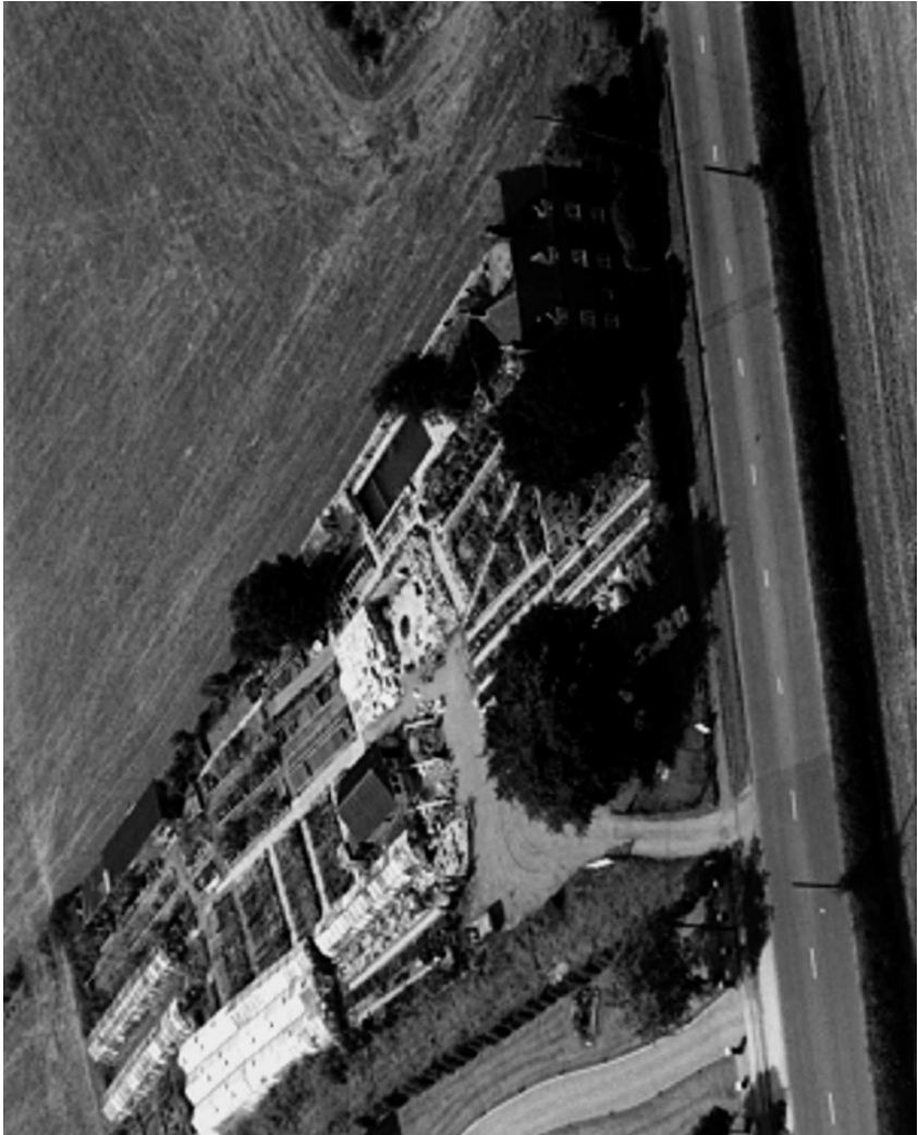
An Aerial View Of The Garden Centre With The New Glass Greenhouses.
